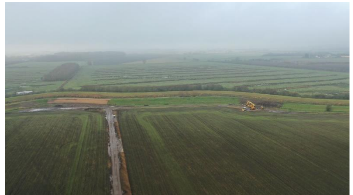
Photograph 2: Drone Image of Barlings Repairs 2020
