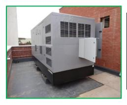
The standby generator was recently delivered and placed on the first floor roof. The generator is a backup source contingency against a loss of mains power when closing the barrier; ensuring that it can be operated as normal should there be a power cut. As a further failsafe there will also be diesel powered emergency power packs to drive the barrier's hydraulic system in order provide a further level of contingency should both the mains power and the generator fail.
