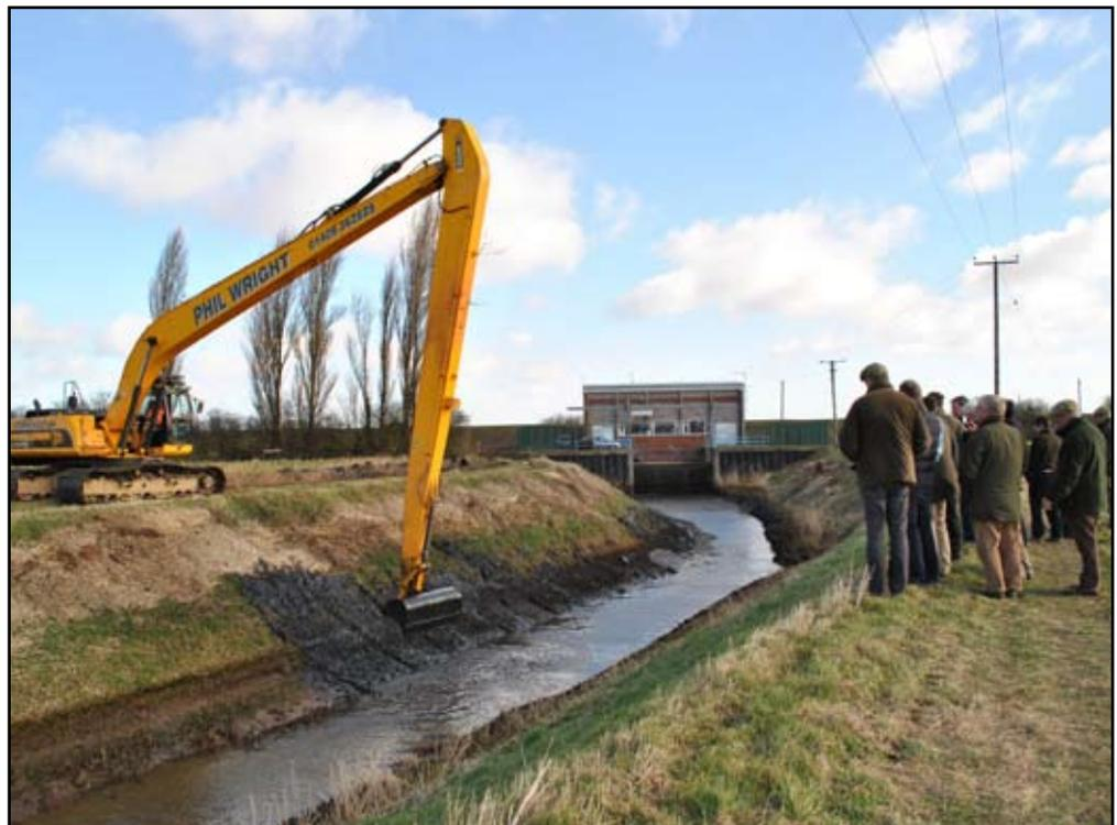
Black Sluice IDB Northern Works Committee members watch dredger operator Kev Methley at work with the 33-tonne, 25-metre reach JCB JS330 machine at Wyberton Marsh
