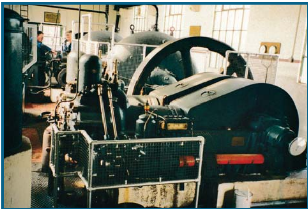
2: QUINCEY'S PUMPING STATION , Culvert Road, Thorpe Culvert, near Wainfleet, PE24 4NJ
