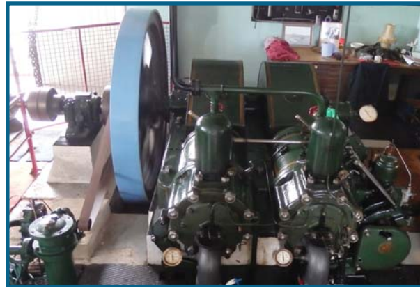
4: TIMBERLAND PUMPING STATION , Walcot Bank, Tattershall Bridge, LN4 4JP
