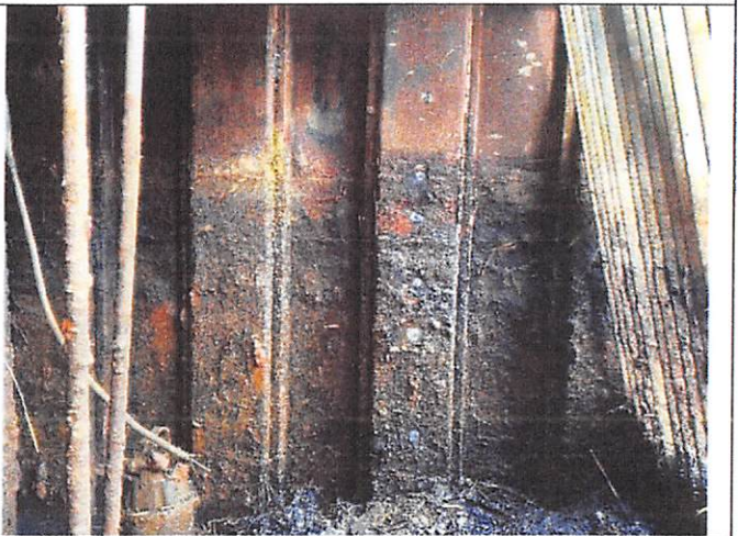
Photograph 04: RHS wall – test area
