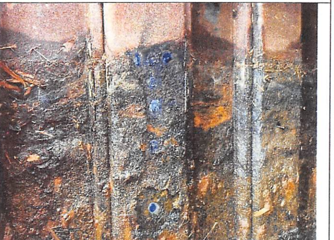
Photograph 06: Test area (wet/dry zone)
