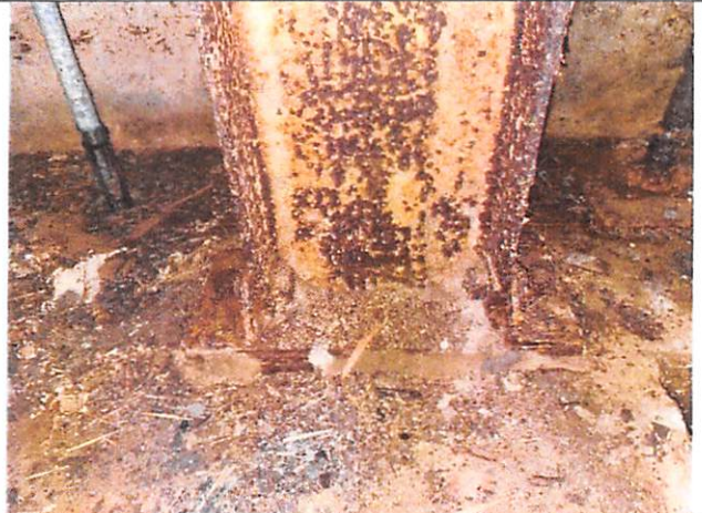
Photograph 8: Stanchion at lower slab level – typical condition
