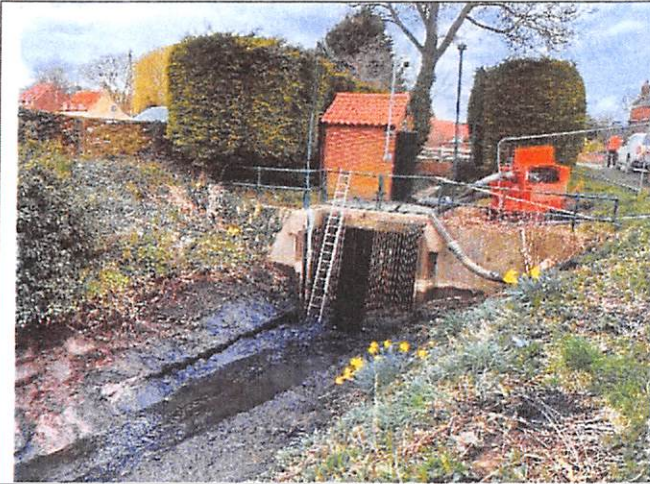
Photograph 01: Pumping Station Intake
