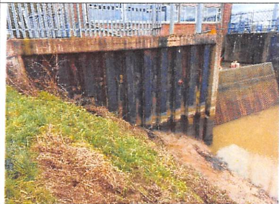
Photograph 3: LHS wing wall – test area
