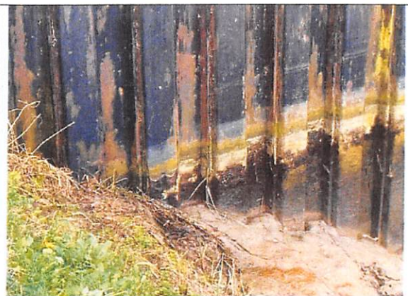
Photograph 2: LHS wing wall – test areas
