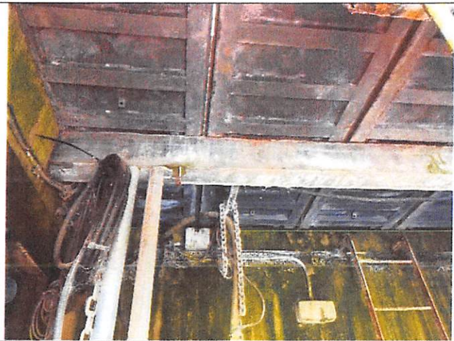
Photograph 03: Galvanised steel support beam (typical)
