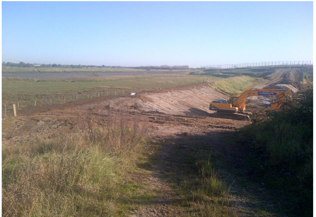
Image: work on the flood bank at Slippy Gowt
