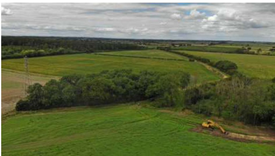
Figure 1: Work starts on the first field swales in July 2020.
