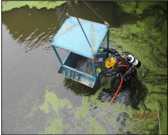
Installation of upstream stop logs and de-watering
