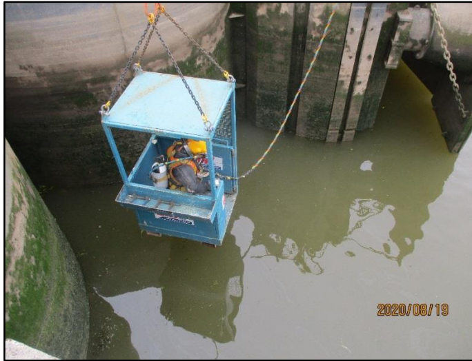
Installation of downstream stop logs
