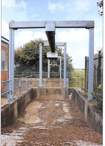
The weedscreen cleaner was installed in 1999, and this scheme is to replace the moving parts to include the trolley and control cabling.
