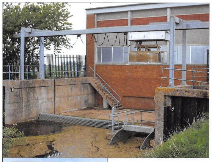
Great Hale Fen Pumping Station maintains water levels to a catchment area of 2,364 Hectares, and has a pumping capacity of 3,482 litres/sec.
