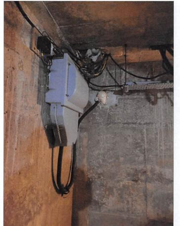
The LV connection, which is below the floor level of the pumping station.
