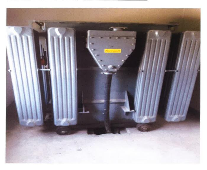
Following a recent inspection of the 9 pumping station transformers, this one at Gosberton pumping station, that also powers Dowsby Fen pumping station, is at point of failure.
